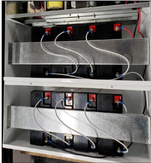
Battery brackets installed on the front
